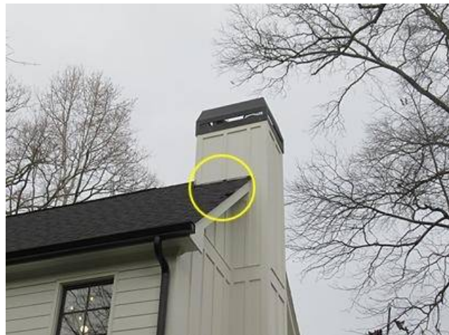
Photo 24-2 BACK LEFT SIDE OF THE ROOF.
