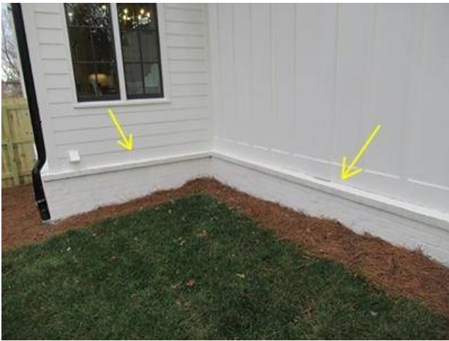
Photo 9-5 BACK RIGHT SIDE OF THE STRUCTURE.
