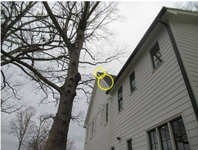
Photo 24-5 RIGHT SIDE OF THE ROOF.
